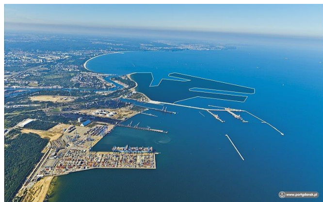
Fig. 1. Outer Port of Gdańsk with newly build container quay. [6]
