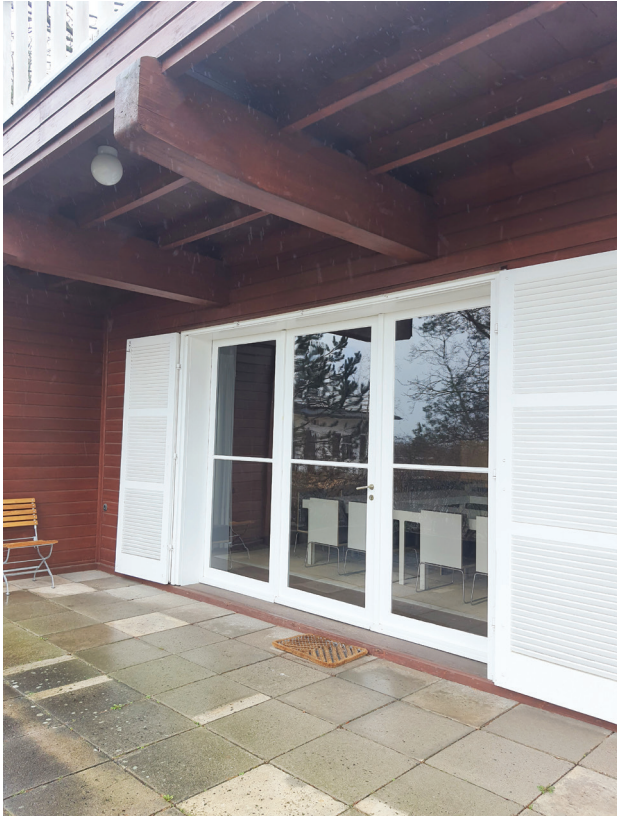
Fig. 4. Einstein's villa in Caputh, protruding beams and large windows in the living room, 1929, architect K. Wachsmann (photo by B. Widera, 2023)
