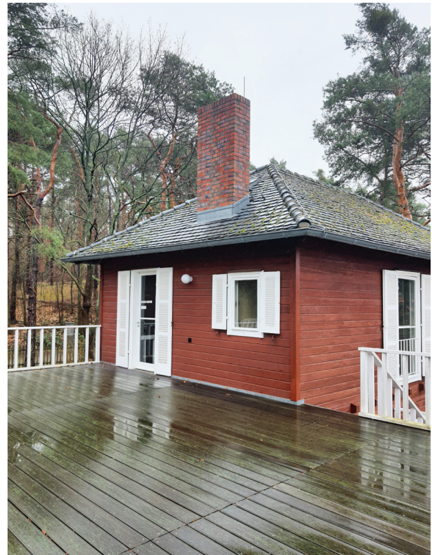
Fig. 3. Einstein's villa in Caputh, view from the north-west, 1929, architect K. Wachsmann (photo by B. Widera, 2023)
