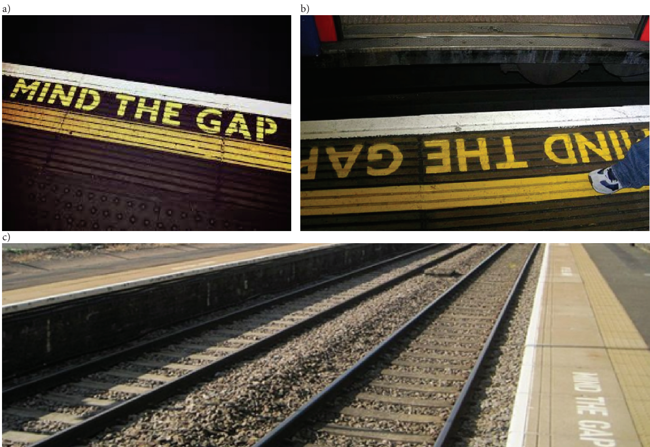
Fig. 22. Character string on platform surface: a) character string readable from the platform (metro) [30], b) character string readable from the coach (metro) [31], c) character string on a railway platform [31]
