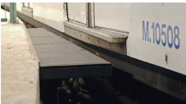
Fig. 13. Footbridge emerging from a platform [1]
