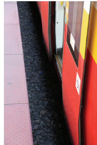
Fig. 4. Enlarged horizontal distance measured between the platform edge and vehicle step in the case of the structure gauge 1-WP [14]
