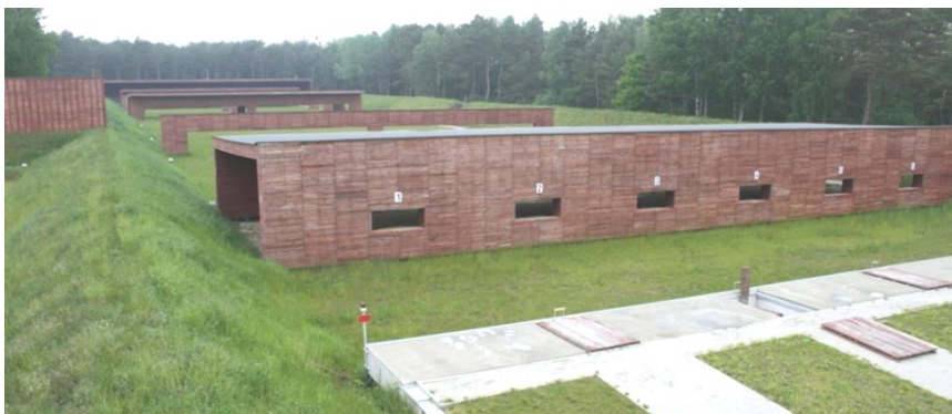
Picture 6. The view of firing zone facilities of 200 m shooting range built in the I-st safety class (9 vertical apertures and main bullettrap roof covering and side protections)
