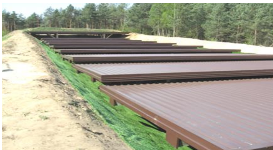
Picture 7. Way for protection of upper firing zone by tilted apertures
