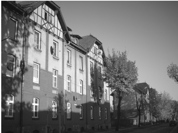
Fig. 4. Buildings in the railway housing estate (author's photo)
