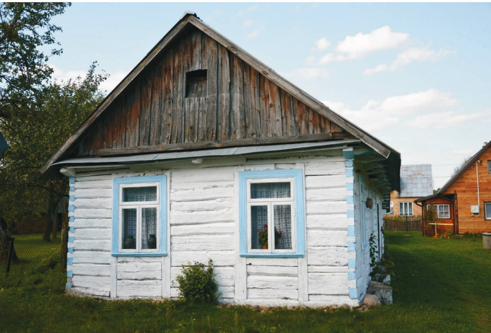
Fig. 13. View of the south wall of the house No. 61, Soce village; photo by the authors, 2017
