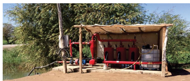
Photo 2. Installation for a drip irrigation system (phot. B. Kulmedov)
