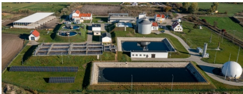
Fig. 2. View of the WWTP in Kościan after modernization
