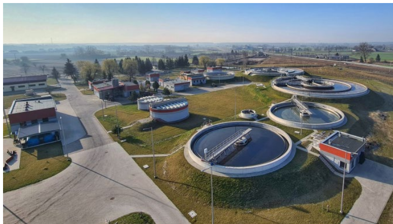
Fig. 1. View of the WWTP in Rawicz after modernization
