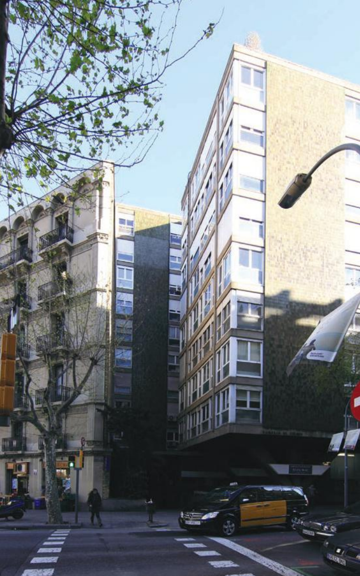
Fig. 12. Antoni Bonet Castellana, Mediterráneo (1966-1967). View of the building with the Cerdà chaflan Photo by author.
