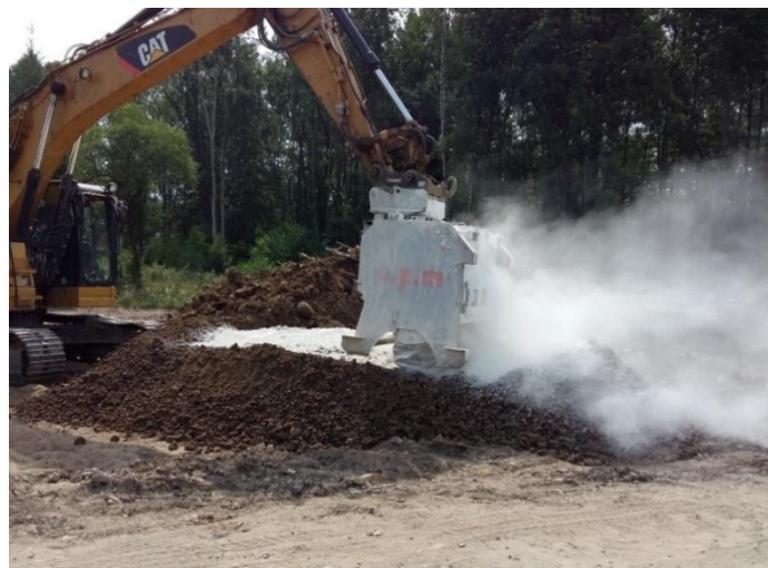
Figure 2. Adding quicklime to the soil using a doser
