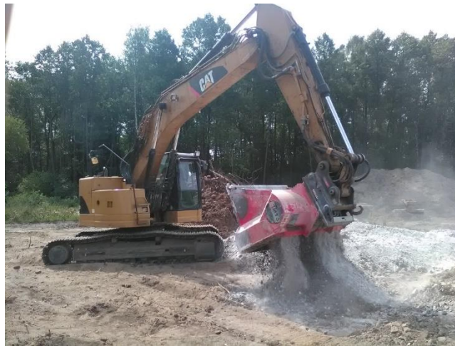
Figure 4. Mixing the soil with lime and further crushing with a recycler
