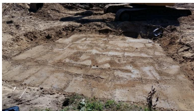
Figure 7. The layer of compacted lime-improved cohesive soil
