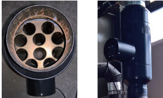
Fig. 6. Construction of the used flue gas – air heat exchanger
