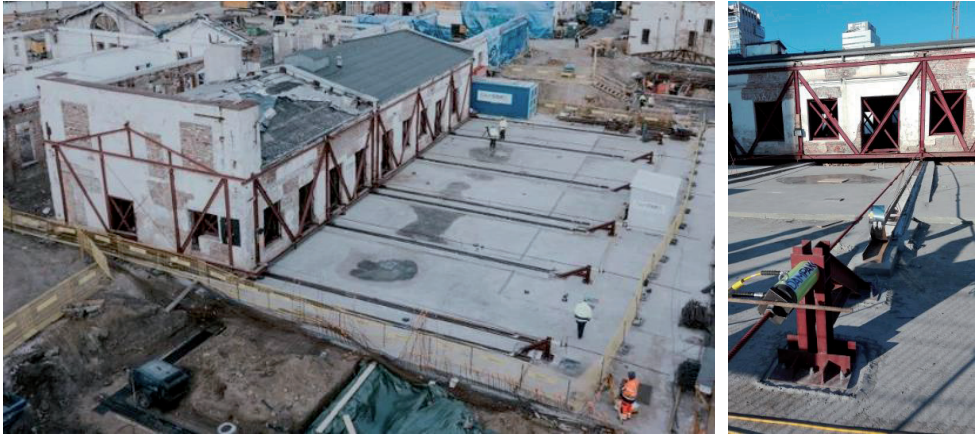
Fig. 9. View of building No. 15 during the operation of relocation
