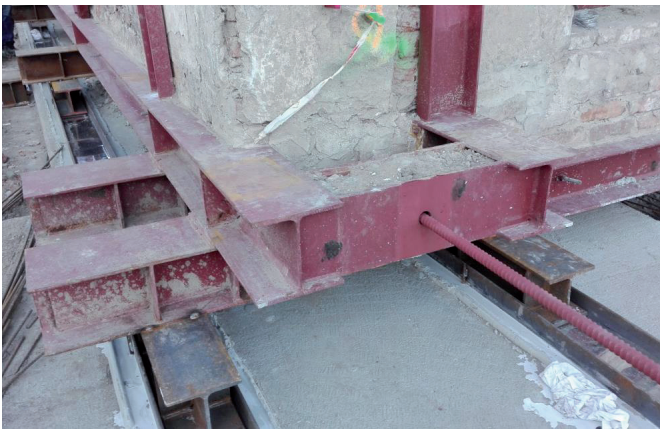
Fig. 8. Outer node of the bottom frame of the stiffening structure of building No. 15; a) design detail; b) erected structure
