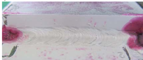
Fig. 3. Results of non-destructive testing of S460N steel joints; a) VT, the specimen W2, the first-laid weld: incompletely filled groove, incomplete fusion; b) PT, the specimen W1 : no imperfections.
