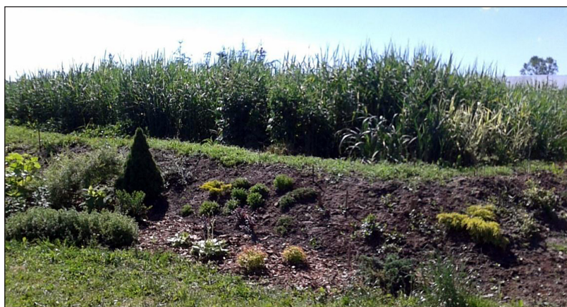
Figure 1. Constructed wetland sewage treatment plant
