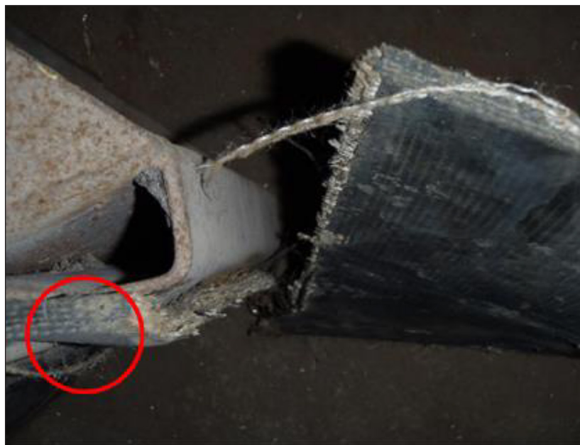
Figure 7. View of the damage location beneath the bucket
