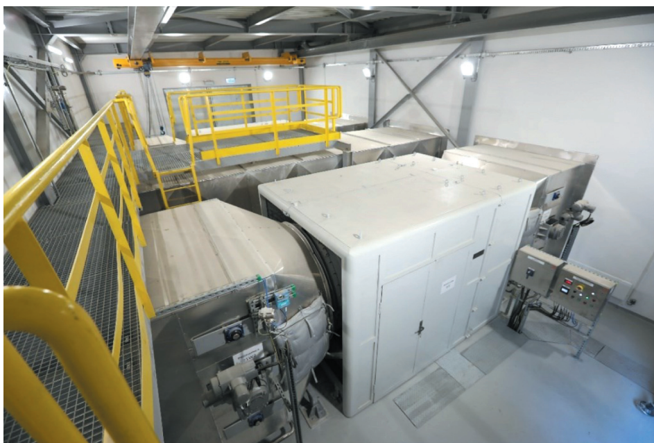
Fig. 5. “Wilson” shaft after retrofitting (phot. R. Stachurski)
