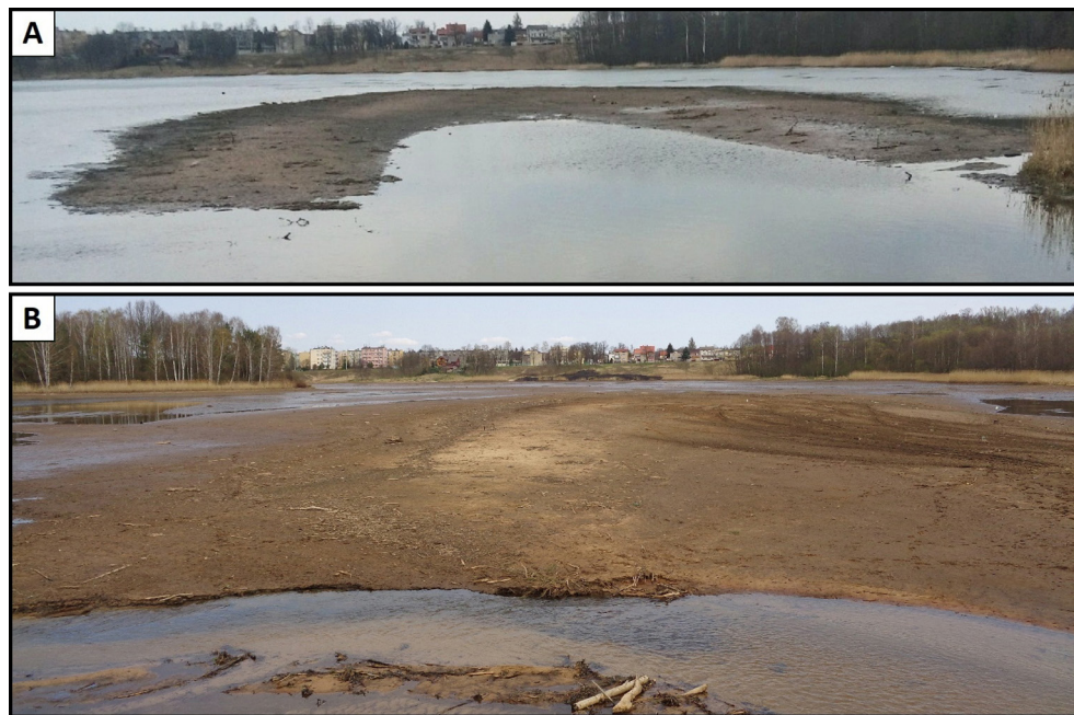
Fig. 5. A - The delta in 2017, prior to reservoir drainage (photograph by S. Piasta); B - The delta in the same year, during hydrotechnical works
