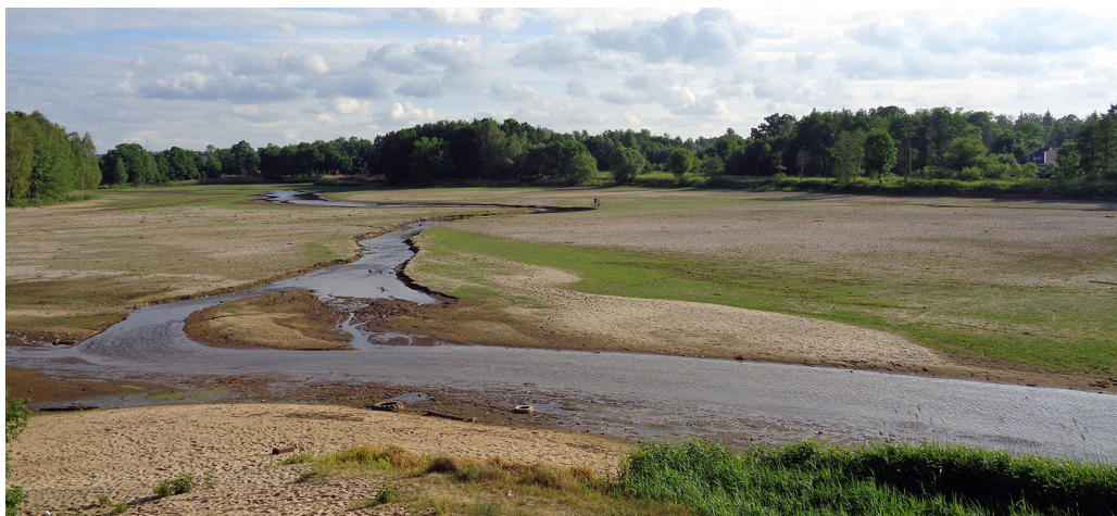
Fig. 3. Dry Suchedniów water reservoir (spring of 2017)
