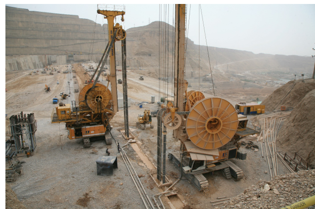
Figure 6: Excavation with BC30 machine alongside the guide wall.
