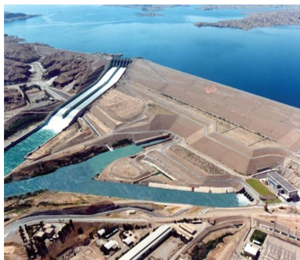
Figure 1: Karkheh Dam, Iran.
