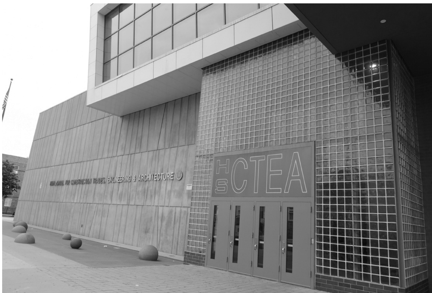
Ryc. 15. High School for Construction Trades, Engineering and Architecture. Fot. autor, 2010
