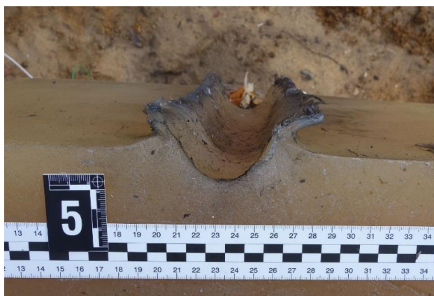
Fig. 7. Damage after a linear charge explosion at a distance of 0 cm.
