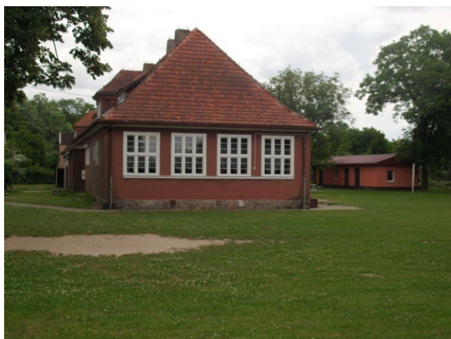
Fig. 5. Polanowice. The 1927 school building (photo by Z. Kuriata)
