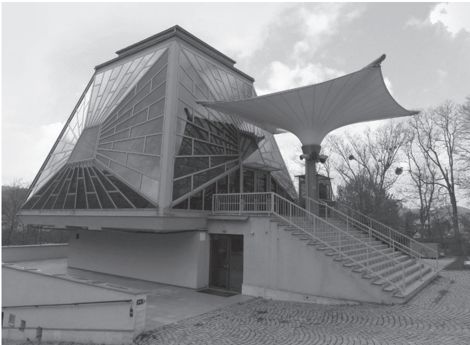
Fig. 4. High-quality architecture ceremony and mourning hall in Vsetín from 1977 with an added roofing staircase, additional heating and cooling of the central glazed space, located at the border of the existing cemetery (photo by K. Frolíková Palánová, 2017)
