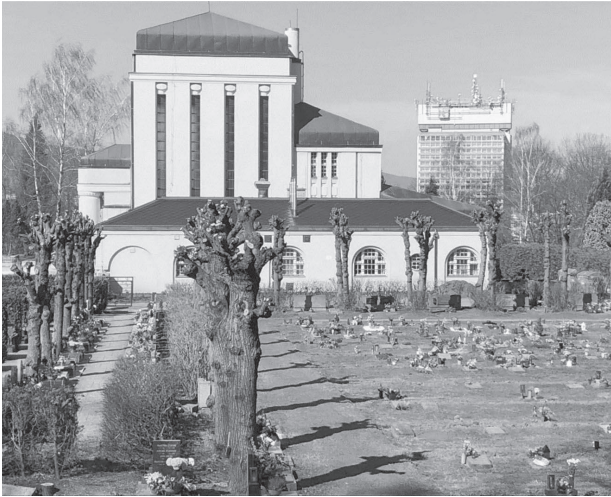
Fig. 2. Crematorium in Liberec (1917) was the first crematorium in Czechoslovakia with an urn garden (photo by K. Frolíková Palánová, 2018)
