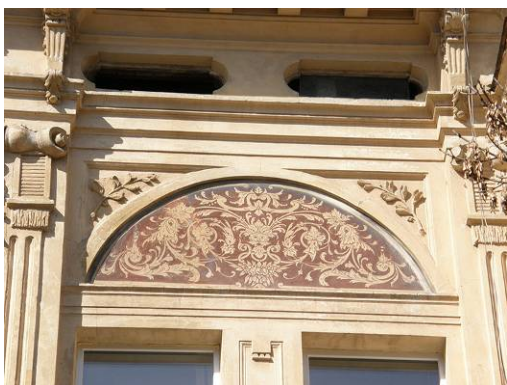
Fig. 7. Fragment of façade painting of the façade of 4 Parkova Street. Imitation of Sgraffito. Source: photo by Tetiana Kazantseva
