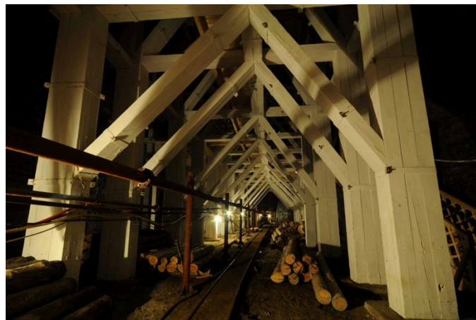
Figure 6: Reconstructed truss-type support in the Gołuchowski cavern in the salt mine Wieliczka (photo ACM)
