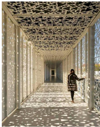
Fig. 3. Implication of new materials and natural ventilation in a porch in the design of a building, od Tripoli avenir design architecture
