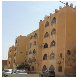
Fig. 5. View of the building units, Biskra, Algeria
