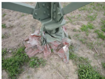
Photo 10. Brush application of coatings
