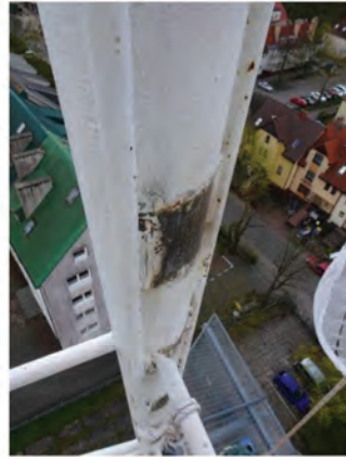
Photo 13. Low surface roughness after cleaning with a grinder (photo: Grzegorz Wasylczyszyn)
