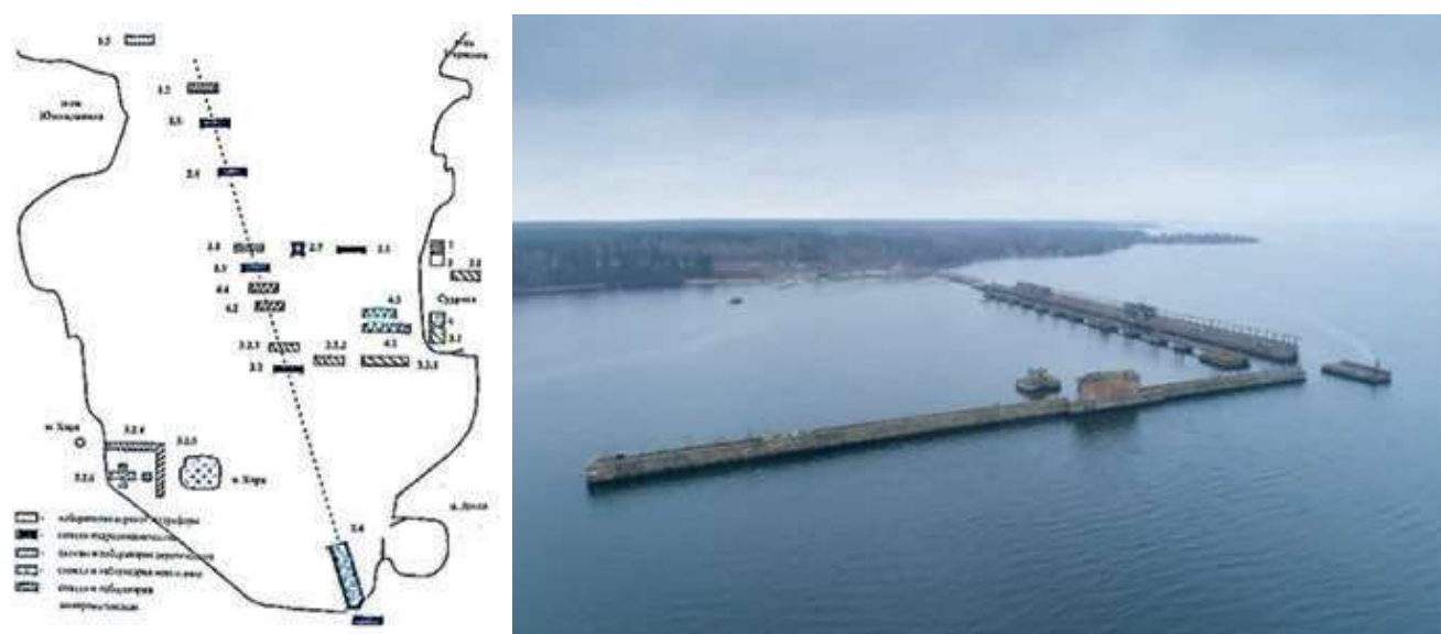
Fig. 2. Plan of the Suurpea Naval Base (Parhomenko, Sazonov), a key element of the Hara Bay navy infrastructure (2003). Photo by Toomas Tuul.
