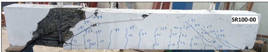
FIGURE 8. Crack pattern for 100% LECA
