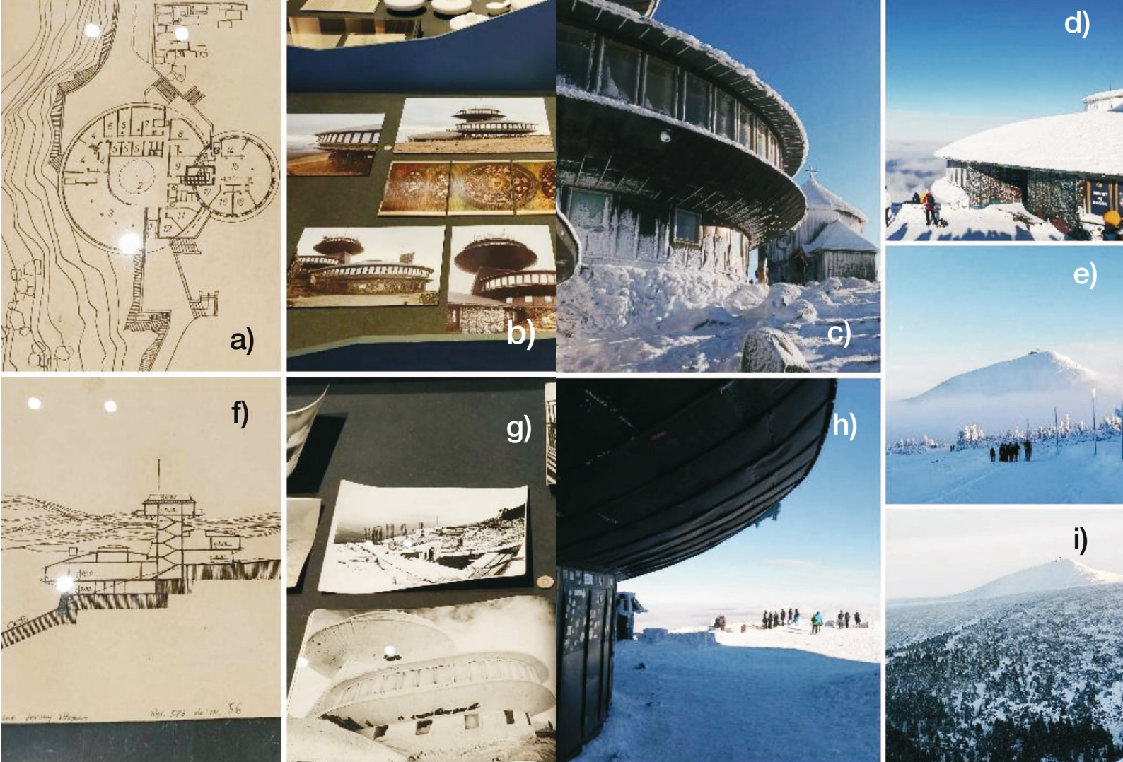
Fig. 8 a-i. High Mountain Meteorological Observatory on Śnieżka – in the past and present: a), f) original drawings of Witold Lipiński and archival materials presented at the exhibition Shape of Dreams – The Architecture of Witold Lipiński ; source: Museum of Architecture in Wrocław 2023, b-e) and g-i) Śnieżka 2022; source: J. Zych 2022
