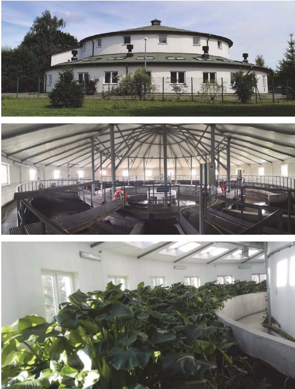
Photo 1. The wastewater treatment plant with activated sludge and hydroponic system
