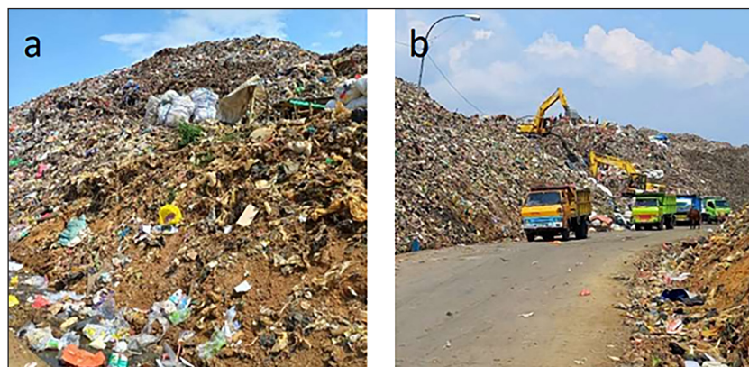
Figure 2. Waste piles in one of the zones in the Makassar City landfill (a), the process of transferring waste from garbage trucks using an excavator (b)
