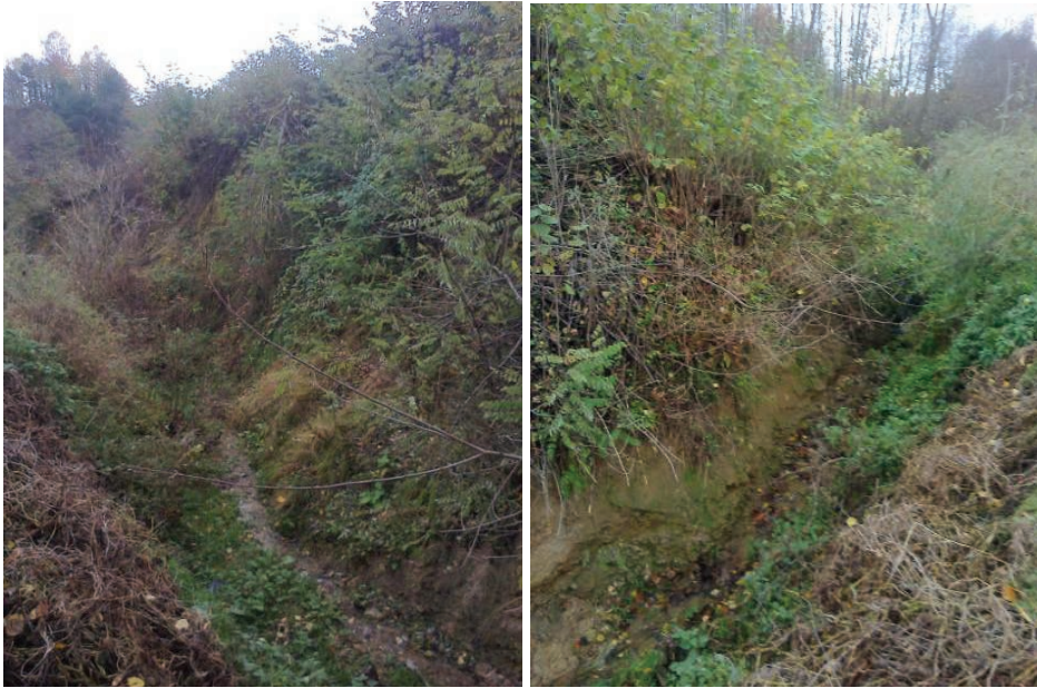
Fig. 3. Example of damages as a result of the water course activity
