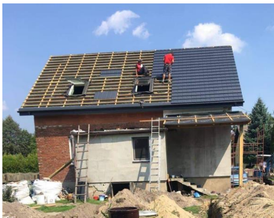
Fig. 2. Roof covering with steel tiles on a wooden frame (Investor's photo, 2020)
