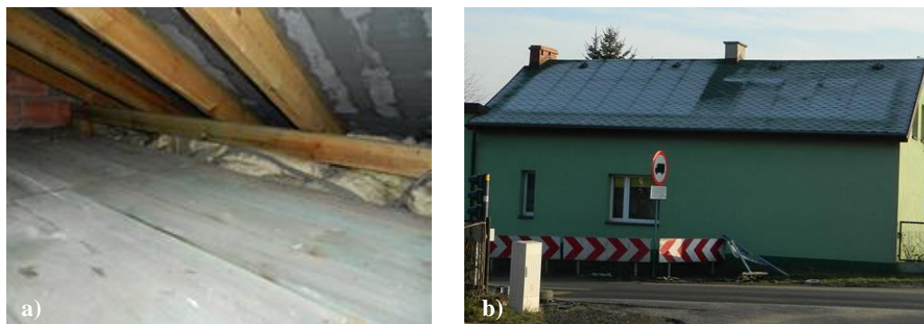
Fig. 1. Between-rafter insulation with mineral wool: a) view of the unused part of the attic; visible stains on the membrane after moisture, b) visible thermal bridges on the frosted roof (own photos)
