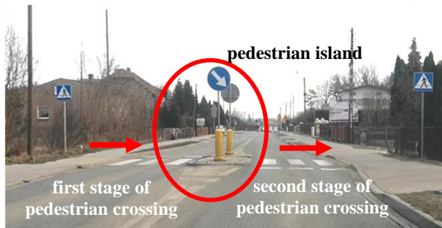
Fig. 10. An example of increasing pedestrian safety through the use of pedestrian islands
