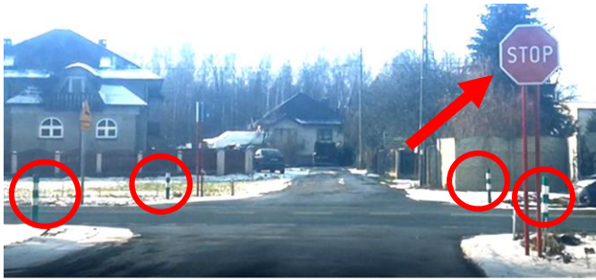
Fig. 6. Incorrect vertical signage at the intersection with a minor road
