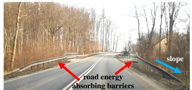
Fig. 9. An example of increasing the safety of vehicle drivers through the use of energy absorbing barriers
