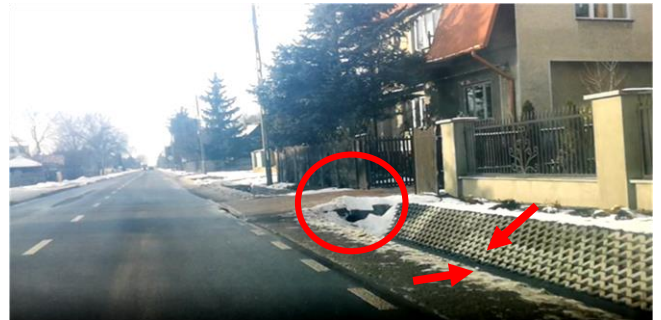
Fig. 8. An example of the correct application of drainage devices
