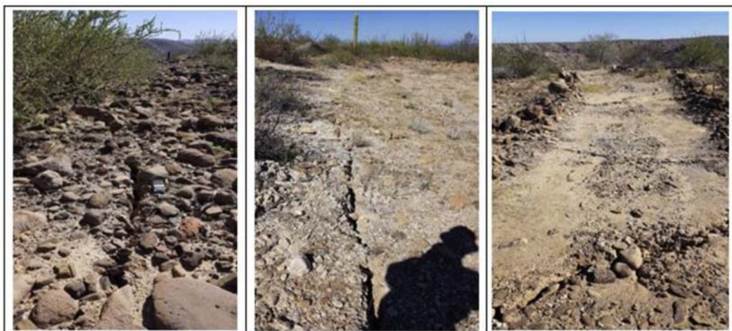
Fig. 4. Observed cracks at M303C.
