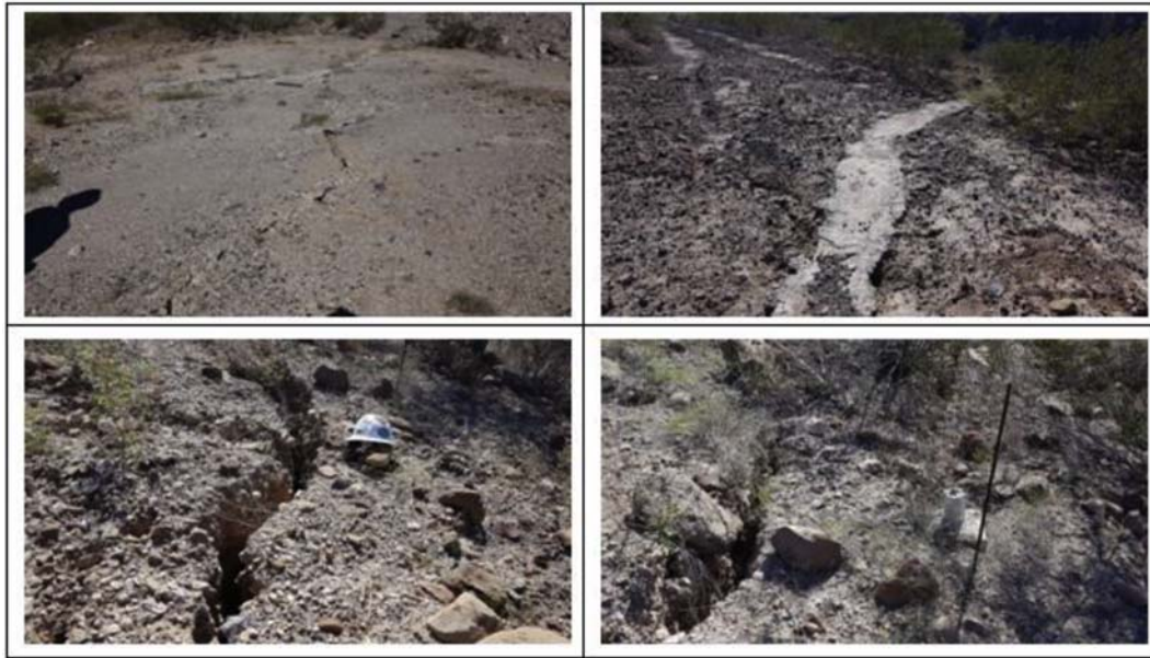
Fig. 2. Observed cracks at M303.
