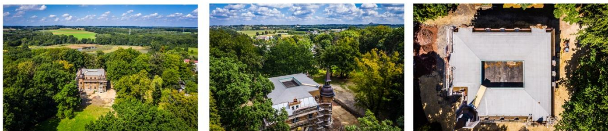
Photo 3-5. Panoramic views of the palace, the roof containing a hidden terrace in the middle and the flat part intended for the photovoltaic panels, 2020 (Author: M. Giba)
