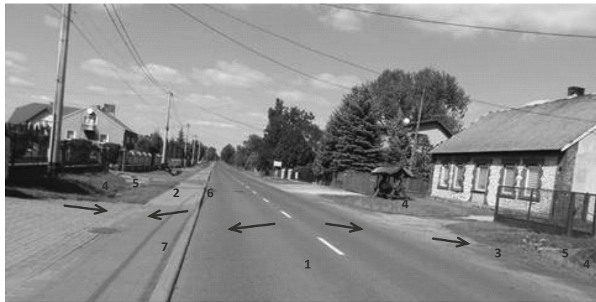
Fig. 1 Drainage devices of exemplary road in built-up area, the arrows show the perpendicular flow directions: 1 - road pavement with roof-like sloping, 2 - sidewalk, 3 - roadside (unpaved), 4 - road ditch, 5 - culvert under an exit, 6 - simple near-curb gutter, 7 - an exit with lowered curb
