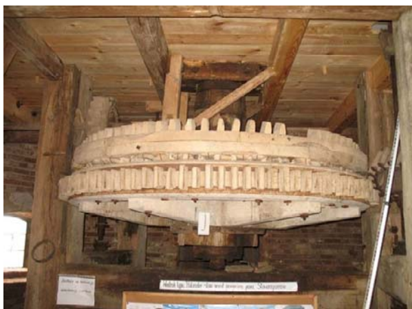
Fig. 3. Łąkorz, the tower mill, the rotating cap zone, relics of the drive mechanism, view from the ground level, present condition. Photo: J. Kielar, July 2011
