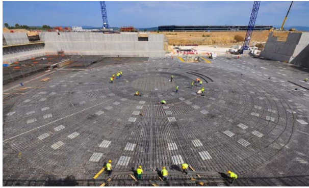
Fig. 9. Construction of the large basement (containing 15 000 m 3 of concrete) for ITER [12].
