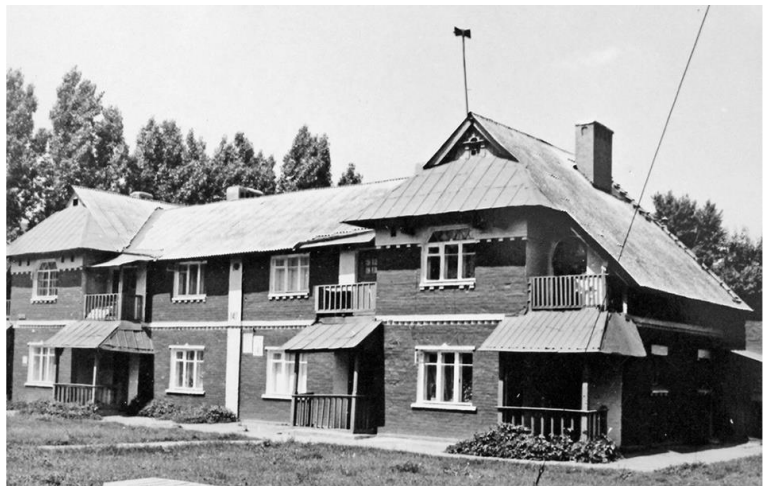
Fig. 3: Typical cottage of the working village in Kharkiv city, 1923. Architect V.K. Trotsenko with the participation of P.Z. Krupko, I.K. Bogomolov, I.G. Taranova-Belozerova. Source: [5]
