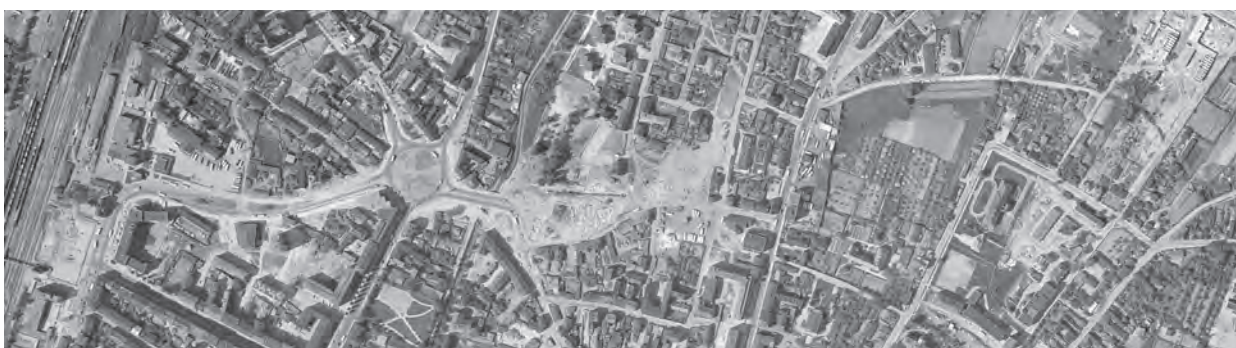
Fig. 10. The beginning of the implementation of the new communication in 1967 Source: Own archive.
