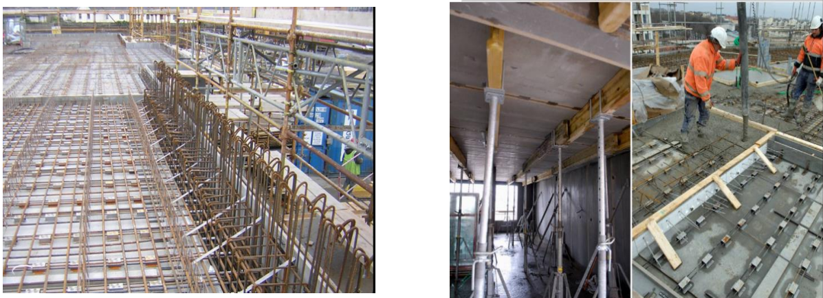
Fig. 1. The application of the VST-system of floor slabs
