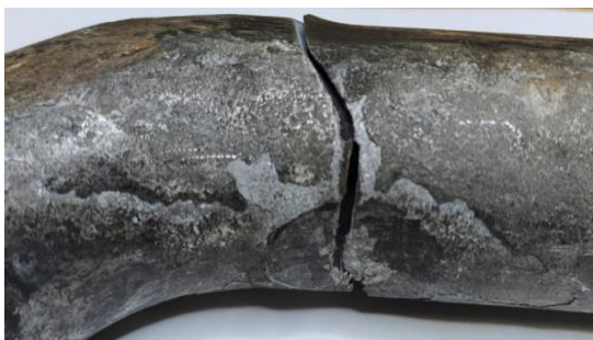
Fig. 10 Ruptured chain link
