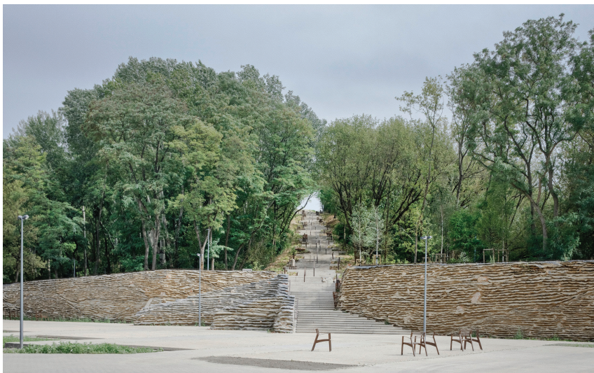
Photo 9. Retaining wall of rubble concrete in the plinth zone of the Mound; source: Michał Szlaga
