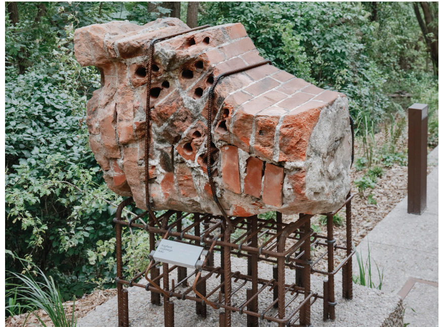
Photo 2. Fragment of a brick arch exposed in the park; source: Michał Szlaga
