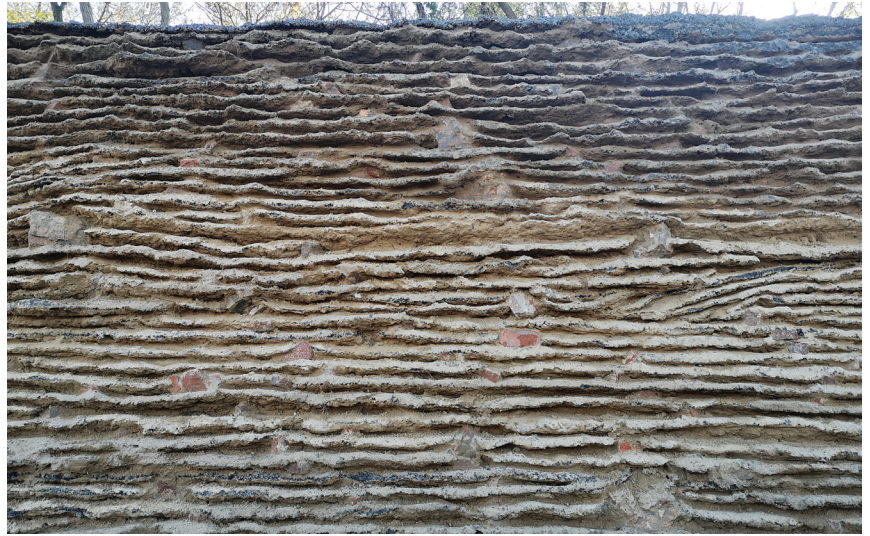
Photo 8. "Geological" texture of retaining walls of rubble concrete. Visible rubble inlaid works; source: Archigrest sp. z o.o. [Limited company]
