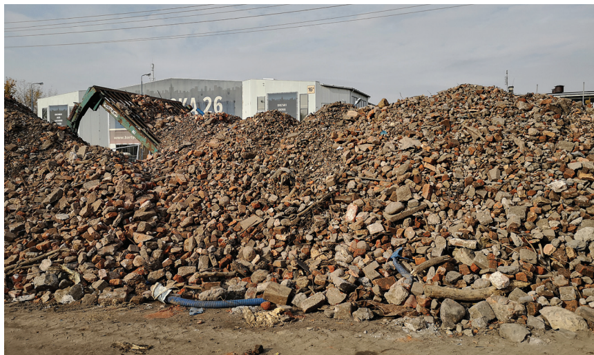
Photo 6. Rubble separated from excavated earthworks, the construction site of the park at Kopiec Powstania Warszawskiego [Warsaw Uprising Mound], 2022; source: Archigrest sp. z o.o. [Limited company].
