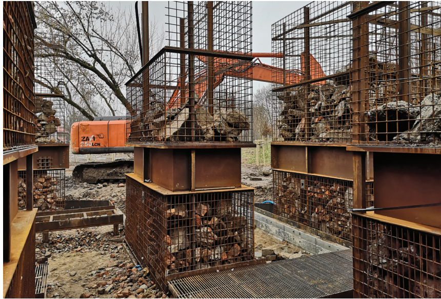
Photo 3. Filling the Lapidarium baskets with rubble during construction works in 2022; source: Archigrest sp. z o.o. [Limited company]
