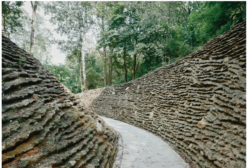
Photo 12. 'Ravine' with walls of rubble concrete; source: Michal Szlaga
