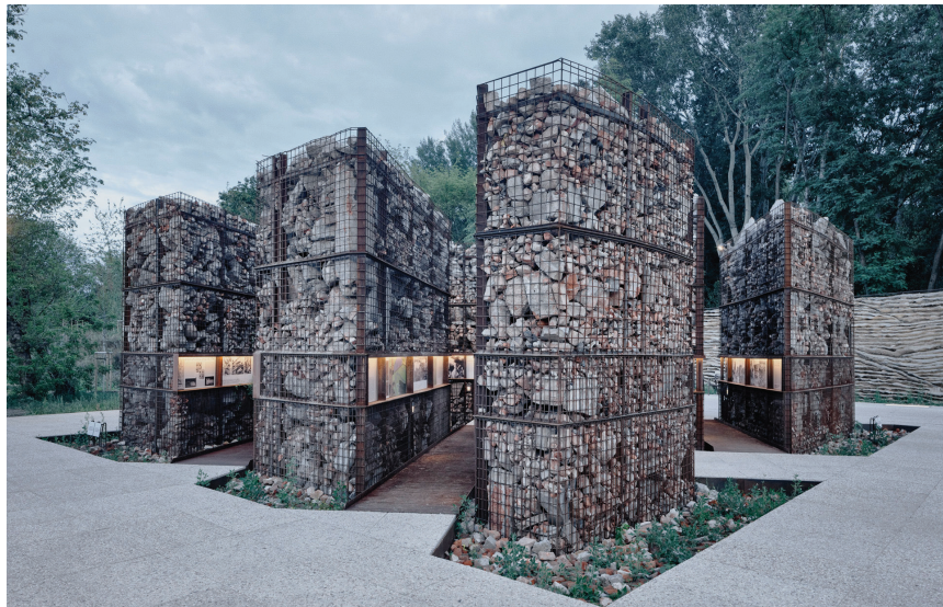
Photo 4. Lapidarium - gabion baskets filled with rubble excavated during earthworks; source: Michał Szlaga
