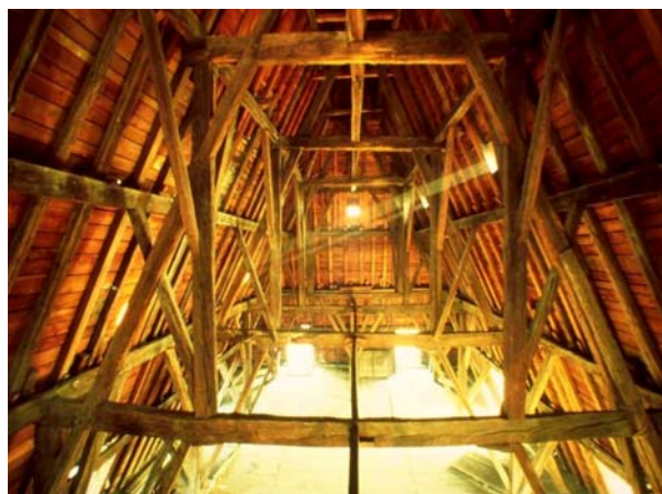
Fig. 33. The timber roof structure of the north-east tower nowadays (photo C.B.)
