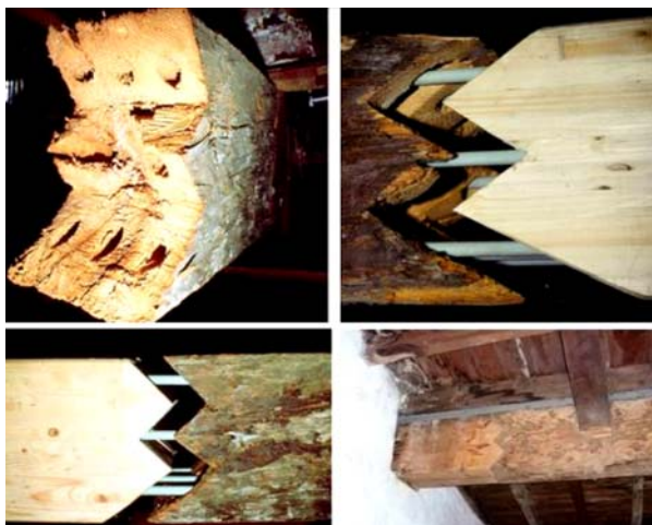
Figs. 14. Reinforcement intervention on tie beams' head-pieces using reinforced glue-laminated timber. Realization (1986)
