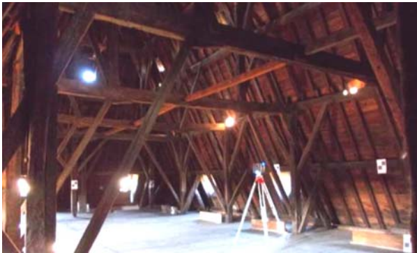
Fig. 21. The Scanner Focus 3D acquiring phase
