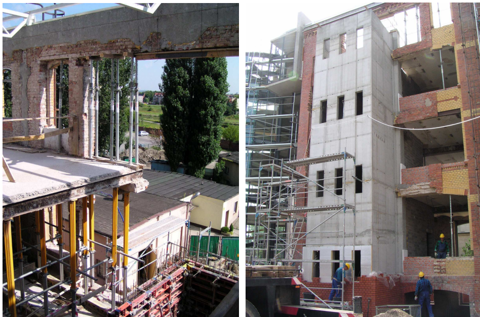
Fig. 16, 17. Restoration of the back staircase basing on SCC concrete
