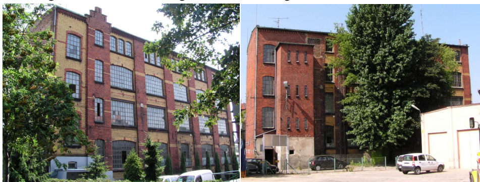
Fig. 1, 2. Dressing room - Bath house before modernisation, the front and back views
