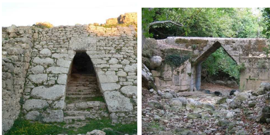
Fig. 7. Left – The needle-vaulted corbelled stone entrance to the ancient Royal Palace in Canaanite Ugarit [W10]. Right – Hellenistic corbelled stone bridge in Eleutherna in the Crete island with a purely triangular shape of a vault [W11]
