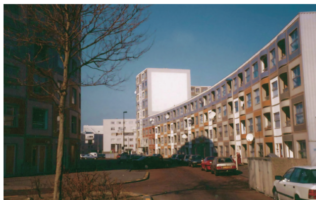
Fig. 3. Large-panel housing construction in the Netherlands (Rotterdam)
