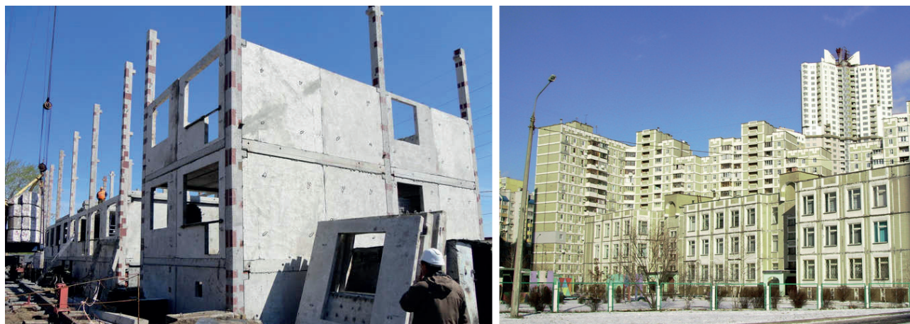
Fig. 1. Prefabricated large-panel systems
