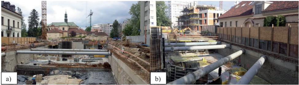
Fig. 2. Implementation of the underground building complex a) construction of the foundation slab, b) construction of the walls and pillars of the underground storey.
