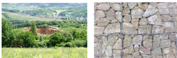
Fig. 5. The Kubo quarry near Malé Žernosky is almost perfectly hidden from human eyes. Quarry stone as one of the products; here the filling of gabions
