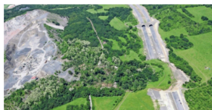
Fig. 7. The 2013 landslide at its largest extent. The thin silvery line represents the damaged and still non-functional railway line [20]
